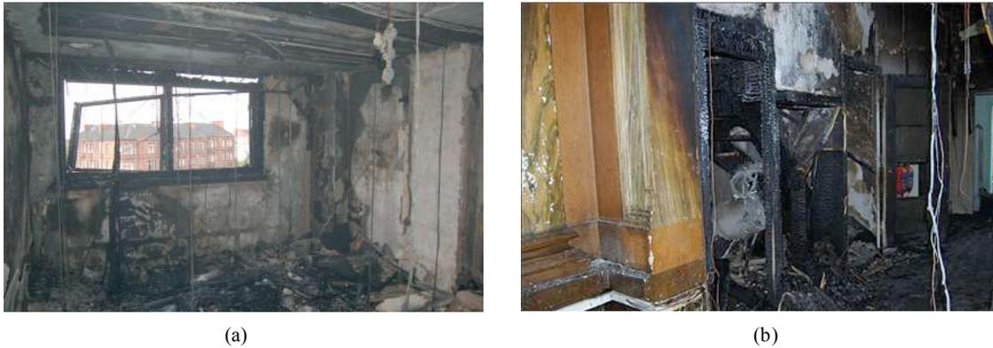
**Figure 1.** Consequences of a fire (a) a post flashover fire with generalized damage [27] (b) a fire that not reached flashover with localized damage (University of Geneva) [28]
