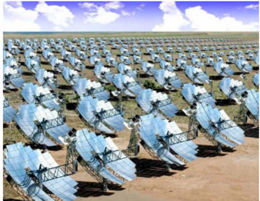
Fig. 4. The Stirling Energy Systems (SES) SunCatcher solar dish farm being developed in California. Each 11.6 m (38 ft) diameter dish automatically tracks the sun and powers a 25 kW Stirling cycle generator. Source: Stirling Energy Systems.
