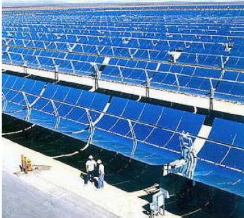
Fig. 3. The Solar Energy Generating Systems (SEGS) solar trough farm at Kramer Junction, California. The concept is that the reflective troughs focus sunlight on a pipe containing oil in a closed-cycle, which heats water to create steam to turbines. In total there are nine SEGS farms, with two at Daggett, five at Kramer Junction, and two at Harper Lake; all in California's Mojave Desert. The total area occupied is 2.4 sq km, generating 354 MW of power. These figures scale up to a footprint of 320 km by 320 km, if we were to supply 15 TW with this method. The nine plants have gradually been installed from 1984 to 1990, demonstrating over 20 years of performance without malfunction. Source: Power Corp.
